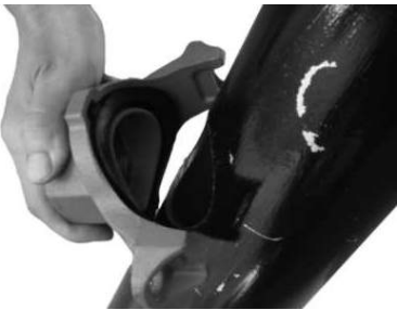
3.Gasket installation Insert the gasket into outlet housing making sure the tab in the gasket line up with the tab recesses in the housing. Align outlet housing over the pipe hole making sure that the locating collar is in the pipe hole.
