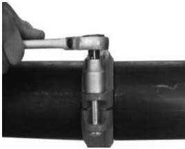
6.Tighten nuts Firstly hand tighten nuts and make sure oval neck bolt completely fits into bolt hole. Then securely tighten nuts alternatively and equally to the specified bolt torque by using spanner.
