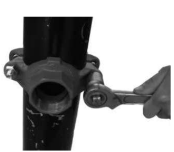
5.Tighten nuts Alternatively and evenly tighten the nuts to the specified bolt torque.
